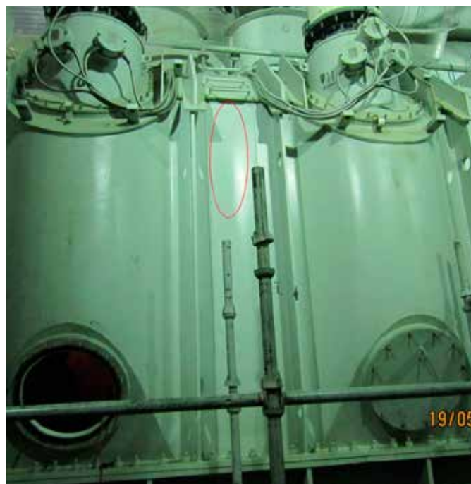
Figure 3: Location of short circuit
